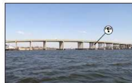
OVERALL VIEW OF BRIDGE
